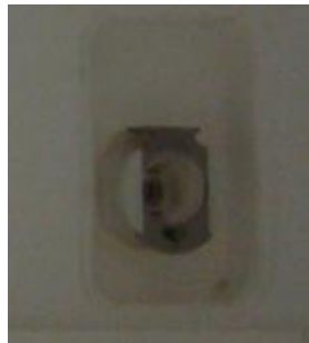
Fig.24 Internal part of vacuum port
